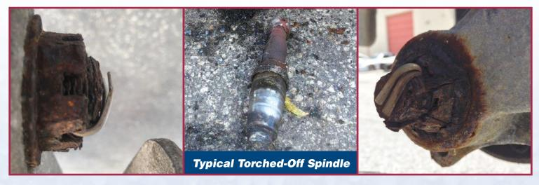
There is now a solution to protect the spindle's castle nuts so they can be removed anywhere at anytime. Tools needed: hammer, pliers, & wrench only
